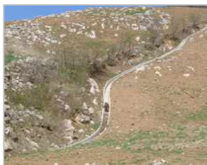
Fig. 4. Example of Diversion Ditch
